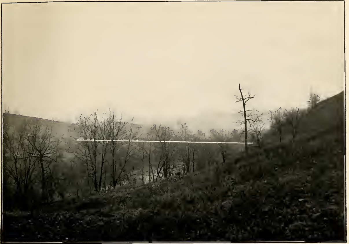
WEST FORK RIVER, W. VA., JANUARY, 1911. View down stream, showing crest of proposed dam.
